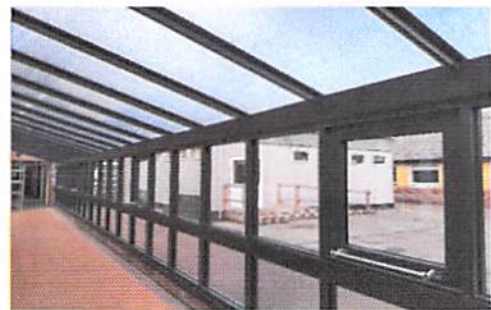
New windows in the B-block corridor
